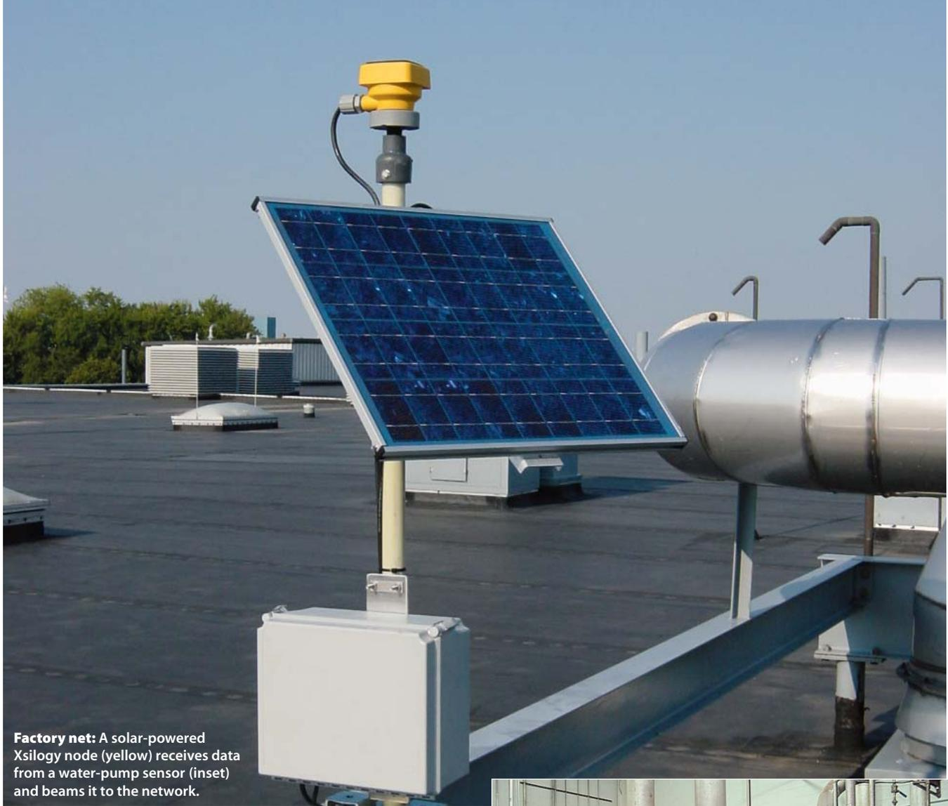
**Factory net:** A solar-powered Xsily node (yellow) receives data from a water-pump sensor (inset) and beams it to the network.
